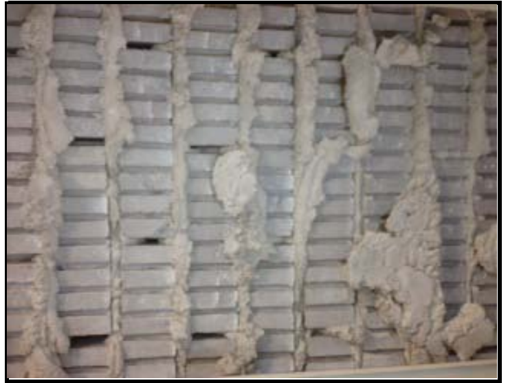
2.) View of remediated areas.
