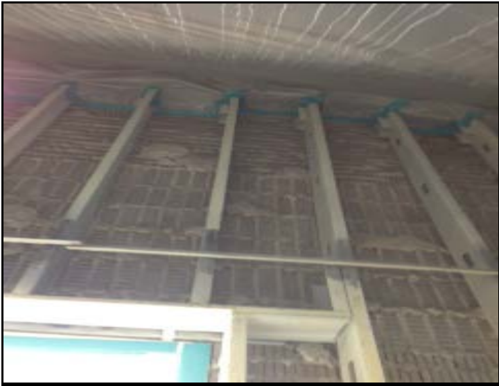
3.) View of remediated areas.
