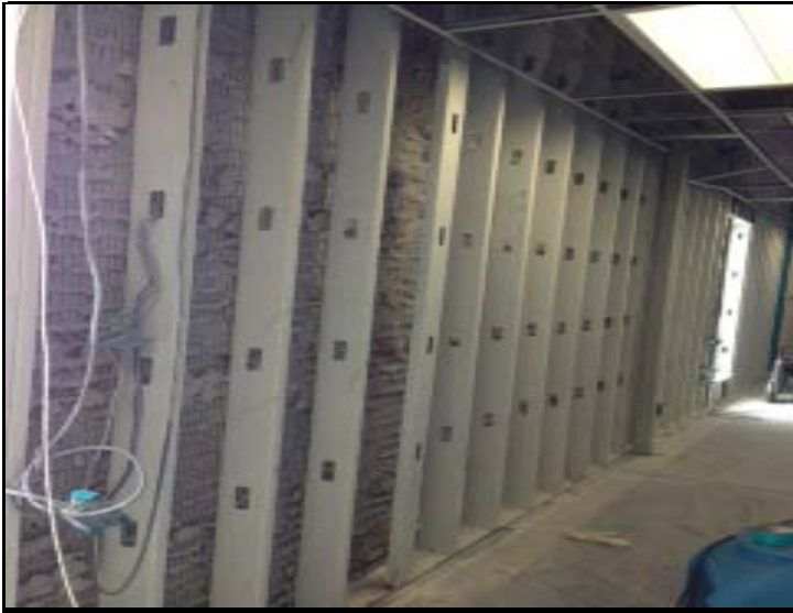
1.) View of remediated areas.
