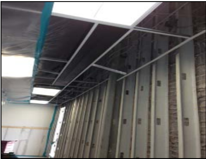
5.) View of remediated areas.
